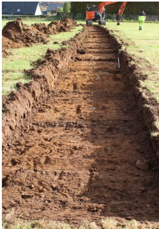
Fig. 35: Trench 11 (Looking East)
